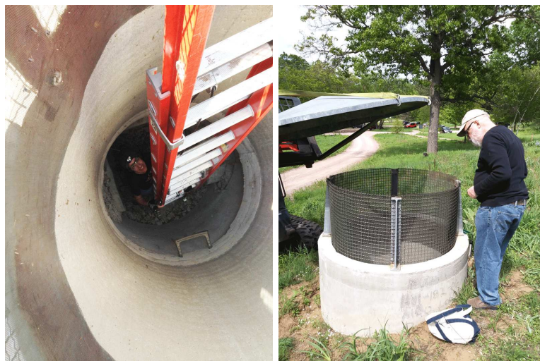
Figure 88. Inside the Manhole, Manhole and the cap
