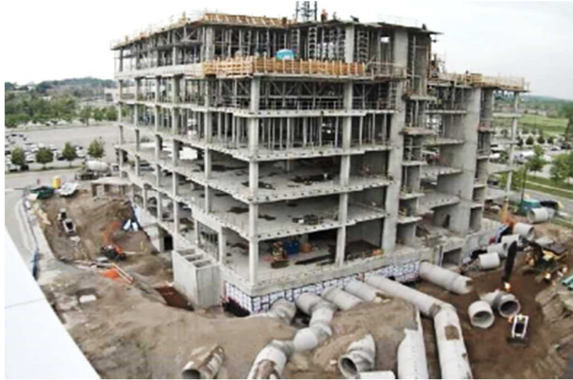
Figure 62. UTSC, Earth Tube Construction 80
