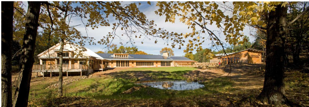
Figure 84. Aldo Leopold Foundation, the Kubala Washatko Architects
