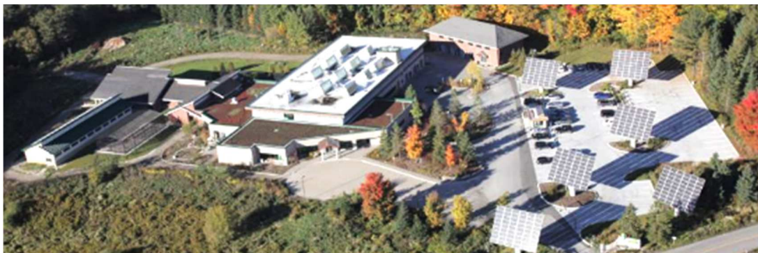
Figure 55. Earth Rangers Centre
