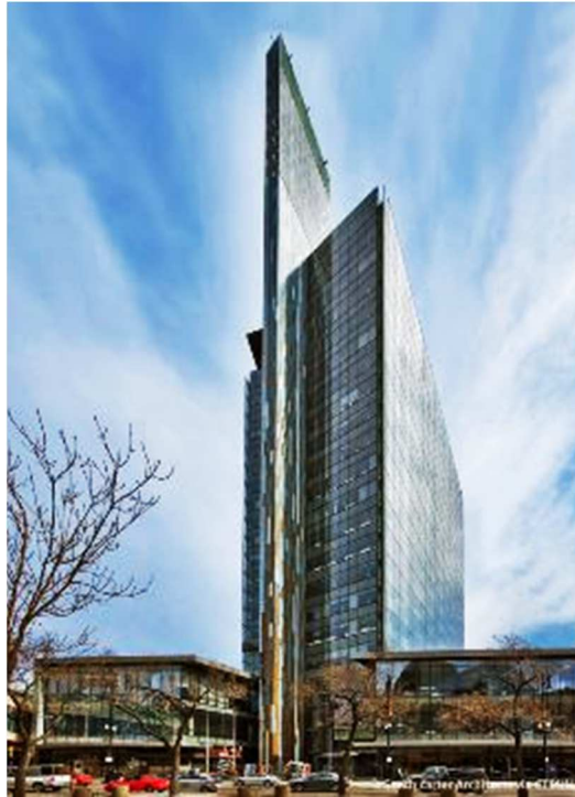
Figure 35. Manitoba Hydro Place 41
