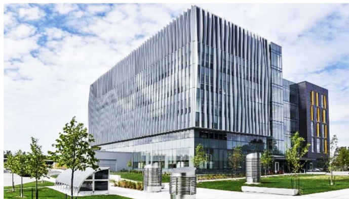
Figure 61. UTSC, Environmental Science and Chemistry Building 75
