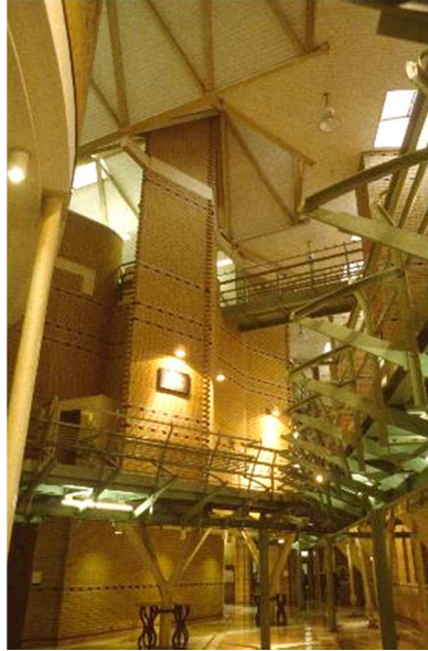
Figure 7. east auditorium exhaust stacks
