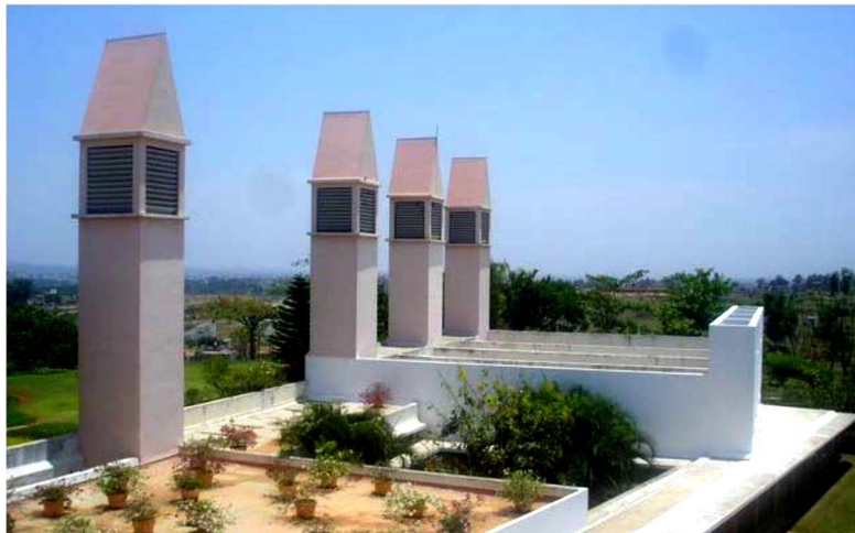
Figure 51. PDEC misting towers
